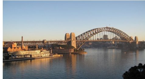
Sydney Harbour Bridge Sydney, Australia
