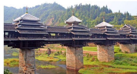
Chenyang Bridge Liuzhou, China
